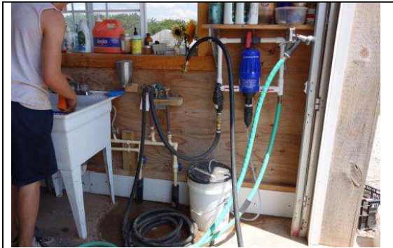
Single use water can also benefit from sanitizer. Sanitizer is not required by the Produce Rule. Many Audits require.
