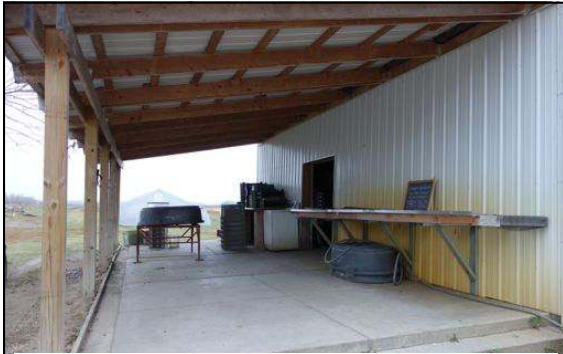
Sloped Floors and Surfaces – Pathogens and flies can breed in standing water.
