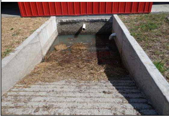
Trap – Straw makes the sediment easier to handle. It will be composted.
